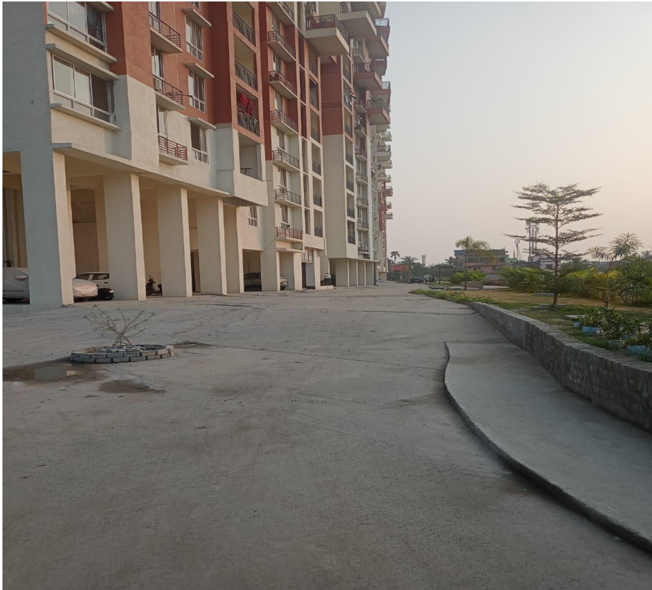
Driveway in front of Block 8-9-10
