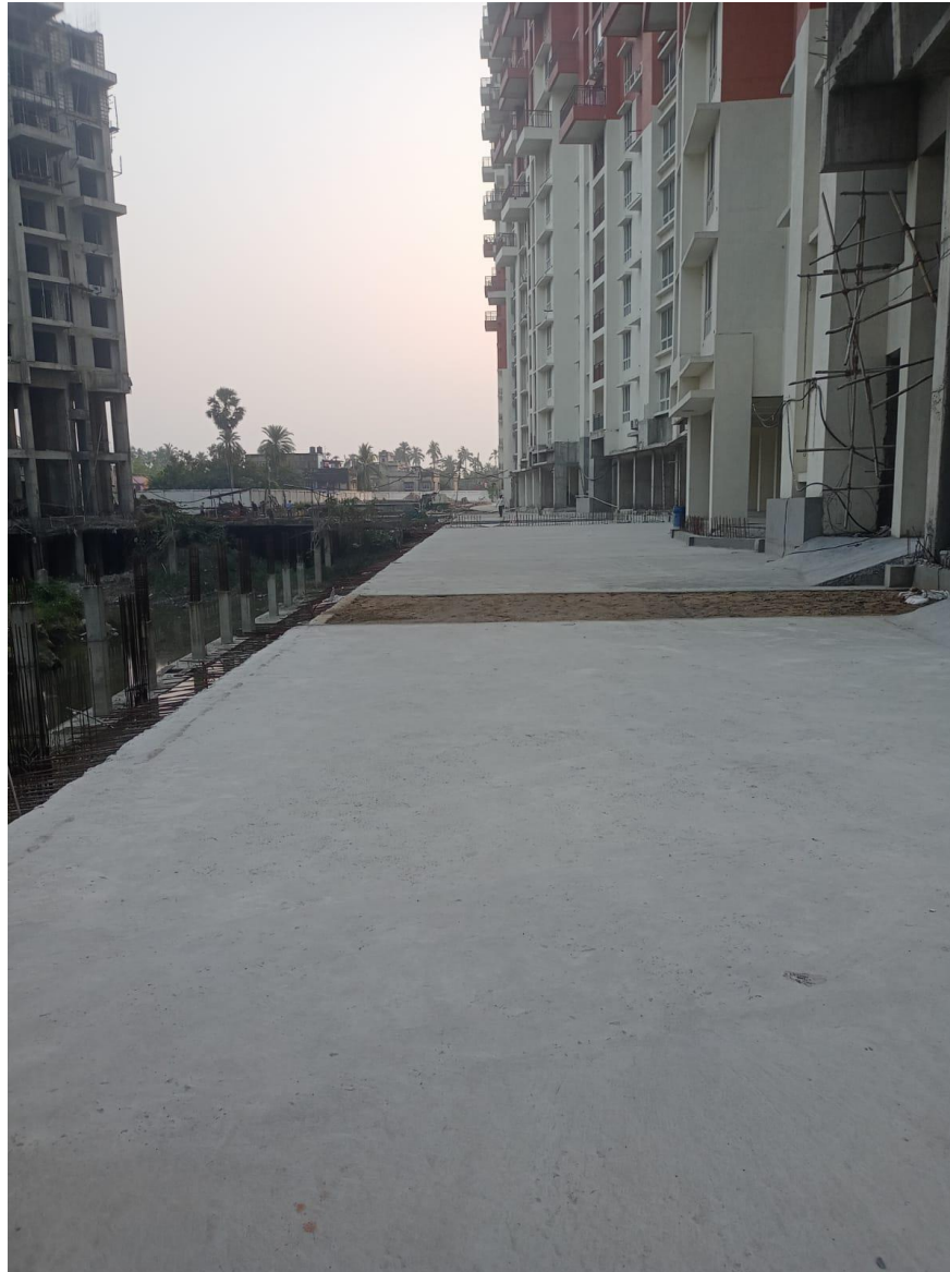
Deck Slab behind Block 8-9-10
